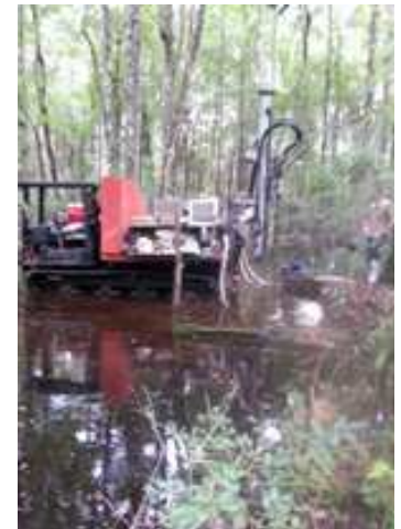
Very Wet Site Conditions
